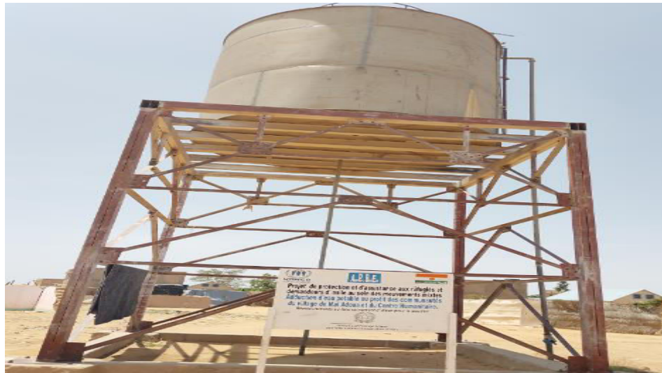
Figure.5 A water tower, August 18 2025. Photograph by Yacouba Magagi.
